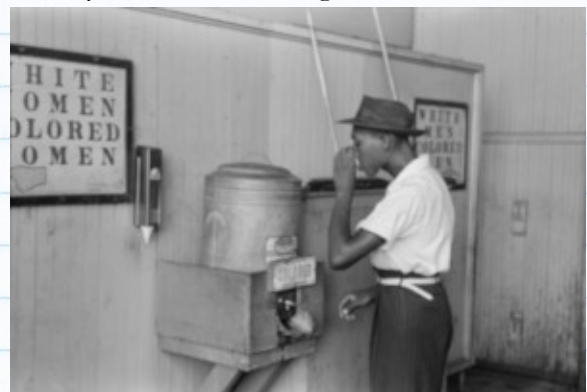
A segregated water station in Oklahoma City
